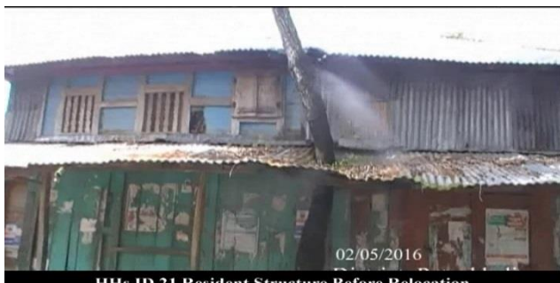
Photo 42: HH 21 before relocation in Polder-43/2C
