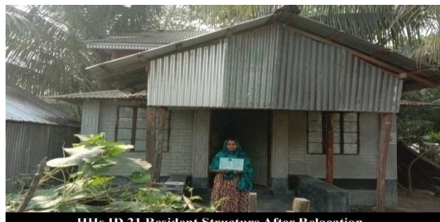
Photo 43: HH 21 After relocation in Polder-43/2C
