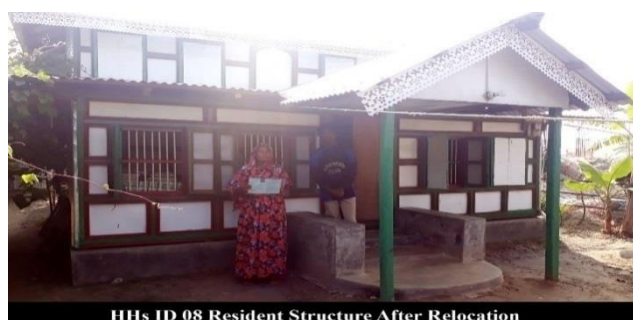
Photo 45: HH 08 after relocation in Polder-48
